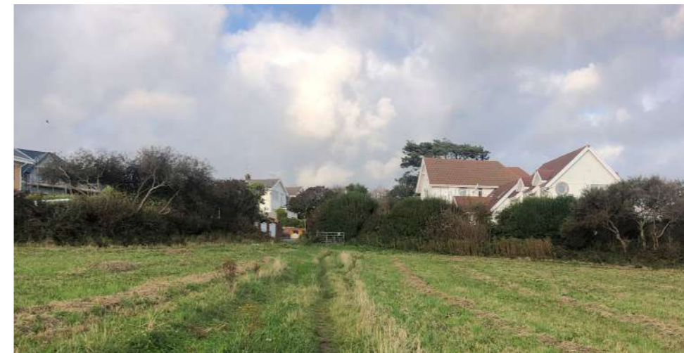
Image showing existing hedgerow and relative levels of the proposed site in relation to property 104 Higher Lane which is at a higher level.
